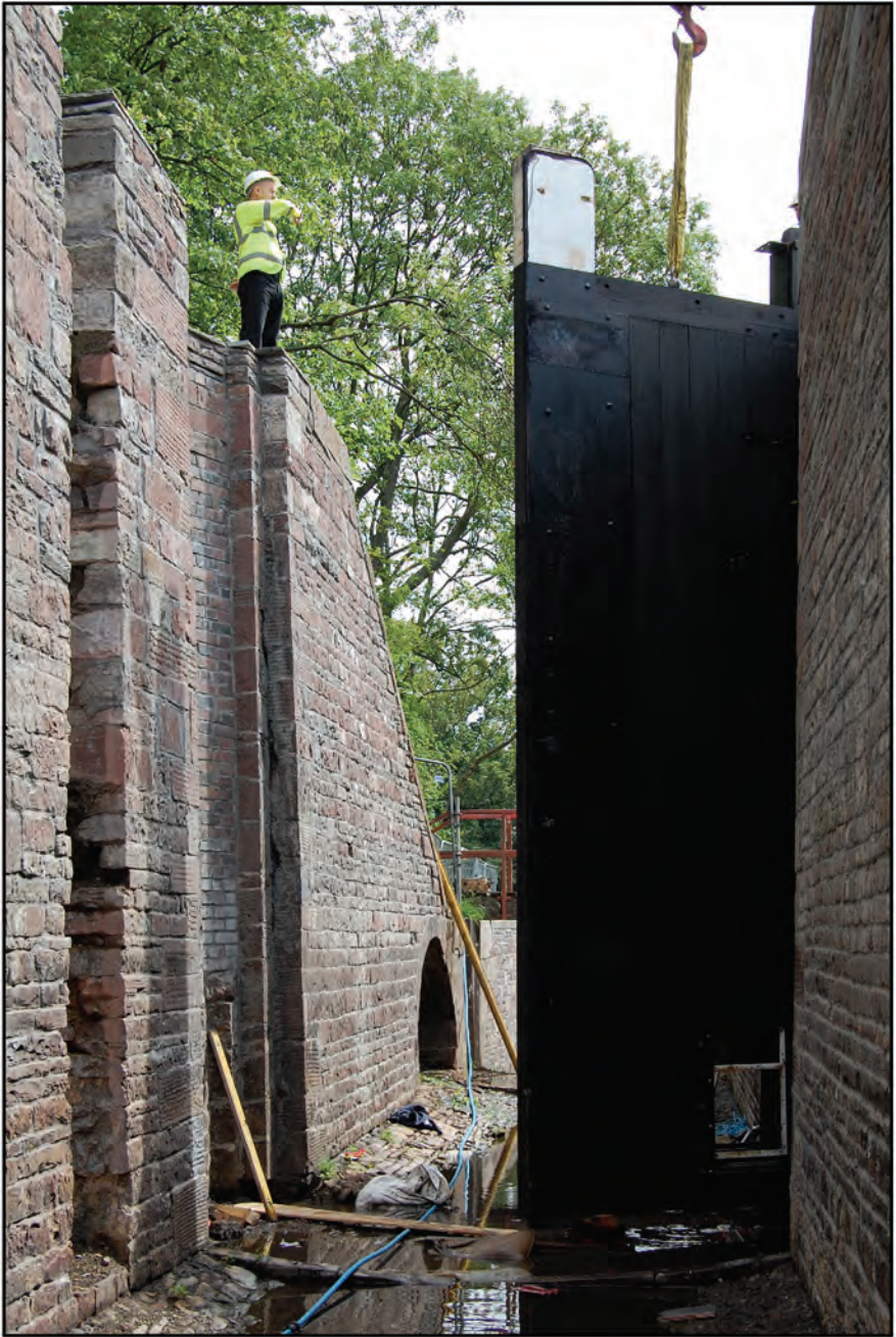
Lock 20 – Installing the first gate, July 2010
