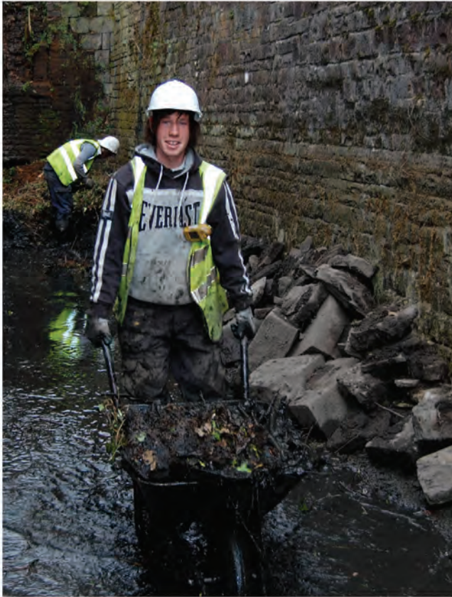
Work begins at Lock 20 – March 2010
