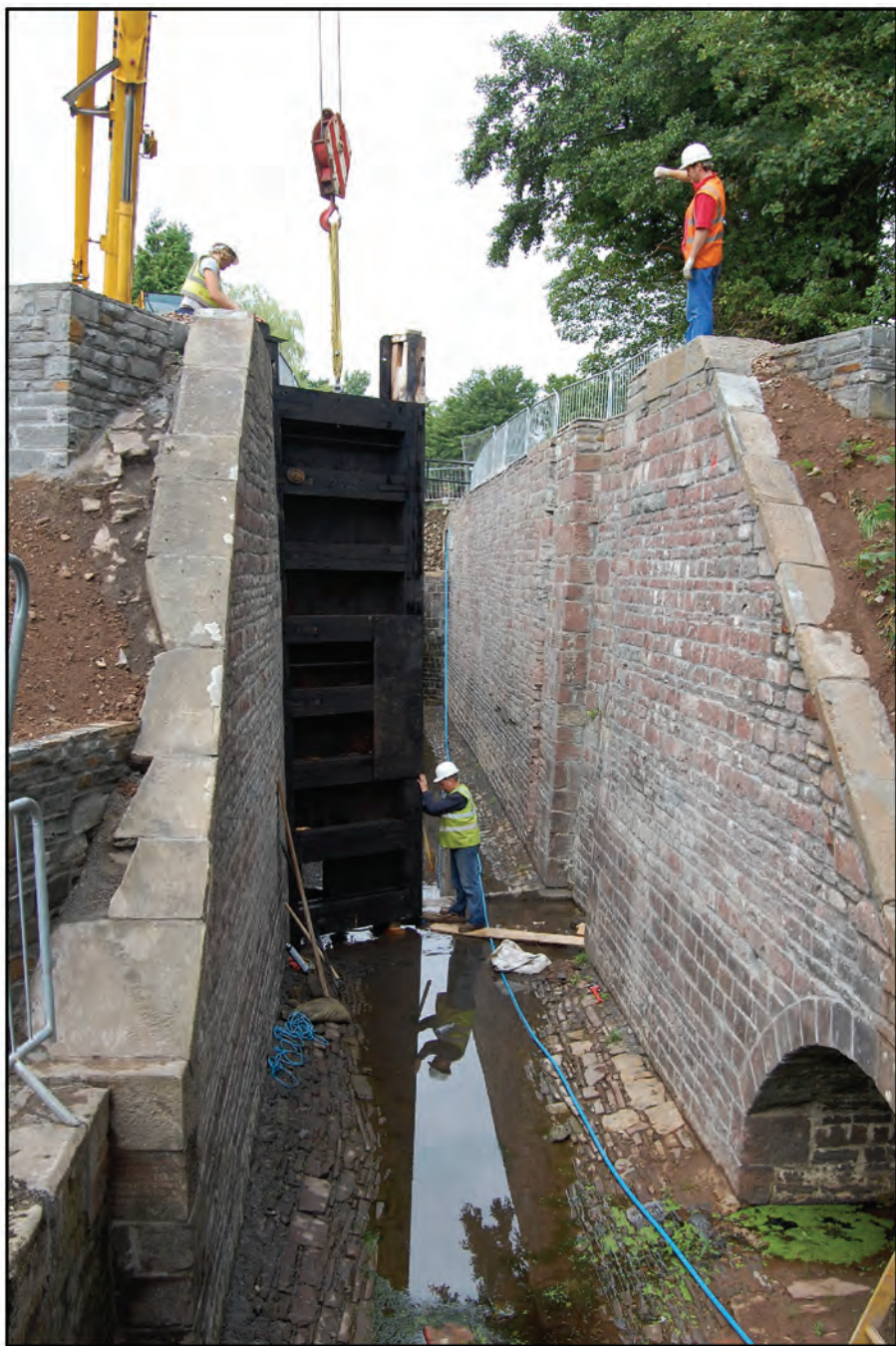
Lock 20 – Installing the first gate, July 2010.
