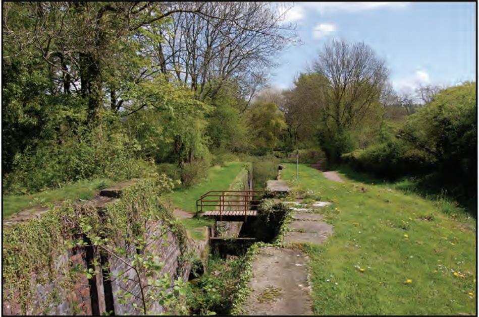
View from Lock 20 – Pre-Restoration May 2009
