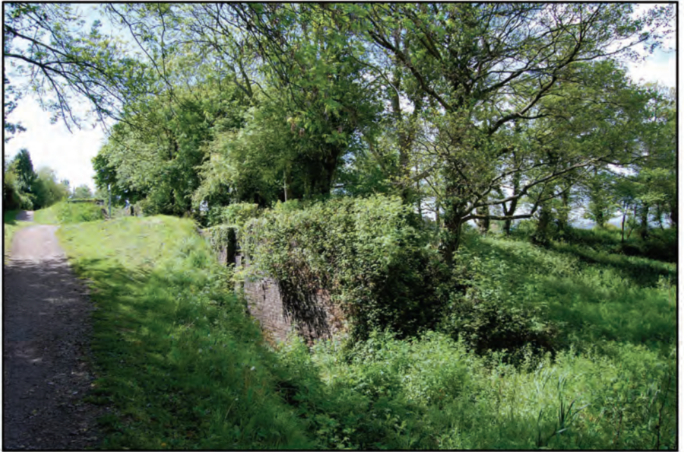
View of Lock 19 – May 2009
